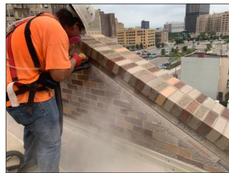
A worker using a respirator while tuckpointing
